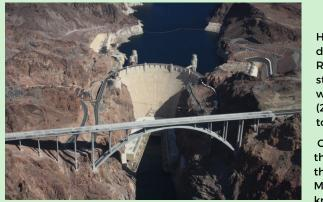
to 45 ft (14 m) at the top. Constructed between 1930 and 1936, it is the highest concrete arch-gravity dam in the United States. It impounds Lake Mead, which extends for 115 miles (185 km) upstream and is one of the largest artificial lakes in the world.
