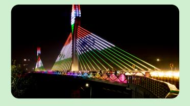
Inaugurated in 2019, Durgam Cheruvu Cable Bridge is a cable-stayed bridge that spans the Durgam Cheruvu lake in Hyderabad. It is suspended by cables from a single pylon that stands 49 metres tall. The bridge's unique design and construction required advanced engineering techniques.
